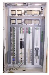
A new electrical room was constructed for the new Motor Control Center (MCC), the new PLC panel, and associated electrical equipment. A new dedicated HVAC system was installed for the electrical room in order to protect the electrical equipment form the harsh environment and to extend the life of the equipment. A new PLC panel was installed along with all new instrumentation and field controls. All electrical and I&C components in the building were replaced.
